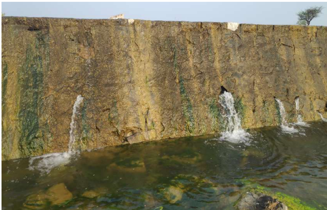
Name of Dam-Kankatrewadi Class-2 Dam Taluka-Khatav, Dist-Satara Defeciency-Leakage through W.W.Bar Date-20.11.2019
