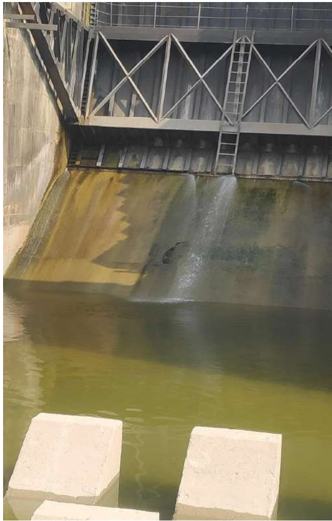
Name of Dam-Ghod Class-1 Dam Taluka-Shirur, Dist-Pune Deficiency-Leakage through Spillway gate Date-08.01.2020
