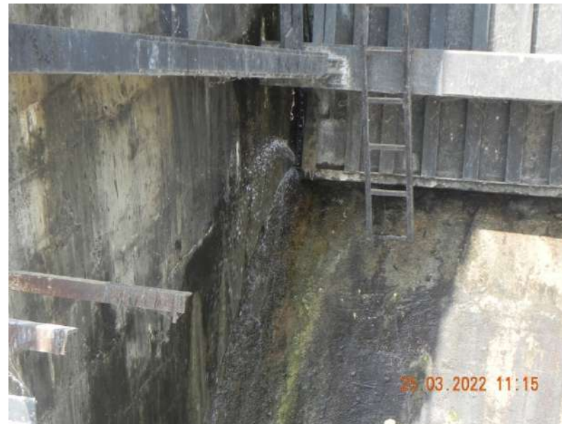
Snapshot -2 Girna Dam (Class II) Tal- Nandgaon, Dist- Nashik Date of inspection:25/03/2022 Leakage through pier near gate is observed.
