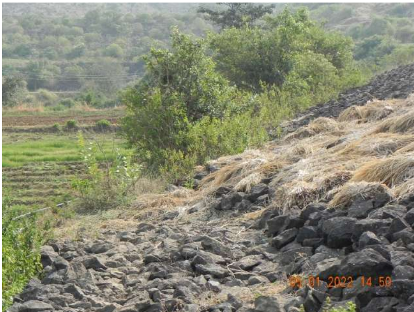
Snapshot-1 Bhegu Dam (Class I) Tal- Kalwan Dist-Nashik Date of inspection:05/01/2022 Rock toe stone is disturbed.(B3)
